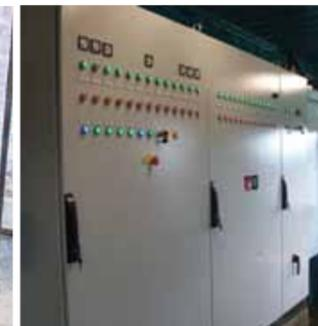
Central control panel for typical large wash spread
